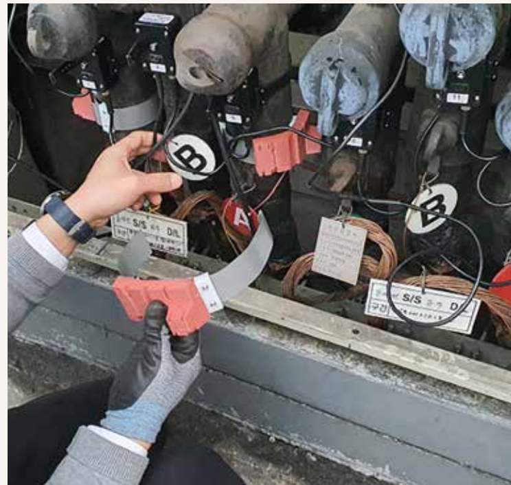
Installation of sensors at elbow connectors in ground switchgear.
