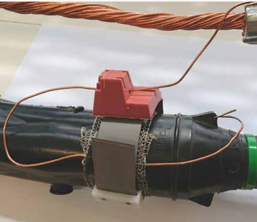
Prototype mounted at cable joint in lab.
